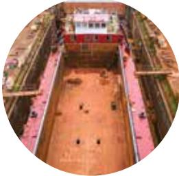
One of the biggest drydocks in Goa's private sector at 84 metres long, 16 metres wide and a draft of 2.5 metres, it has all the necessary infrastructure and facilities to accommodate and repair vessels up to 4000 DWT.
